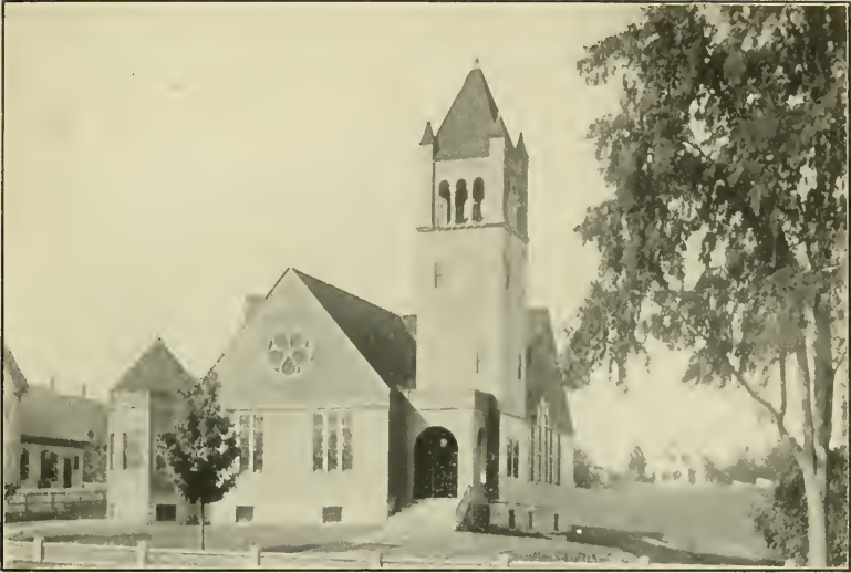
CONGREGATIONAL CHURCH, NORTH CHELMSFORD
